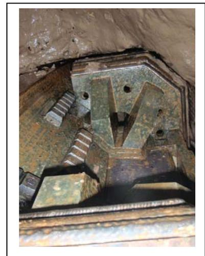
Maintenance and repair under compressed air was performed at up to 5.4 bar air pressure for works at the cutterhead and up to 6.5 bar for works at the stone crusher. Regular compressed air (no mixed gases) and oxygen decompression is successfully in use. In total more than 4.000 h of compressed air works and more than 850 total man interventions are performed. Only 3 minor cases of decompression illness are reported.
